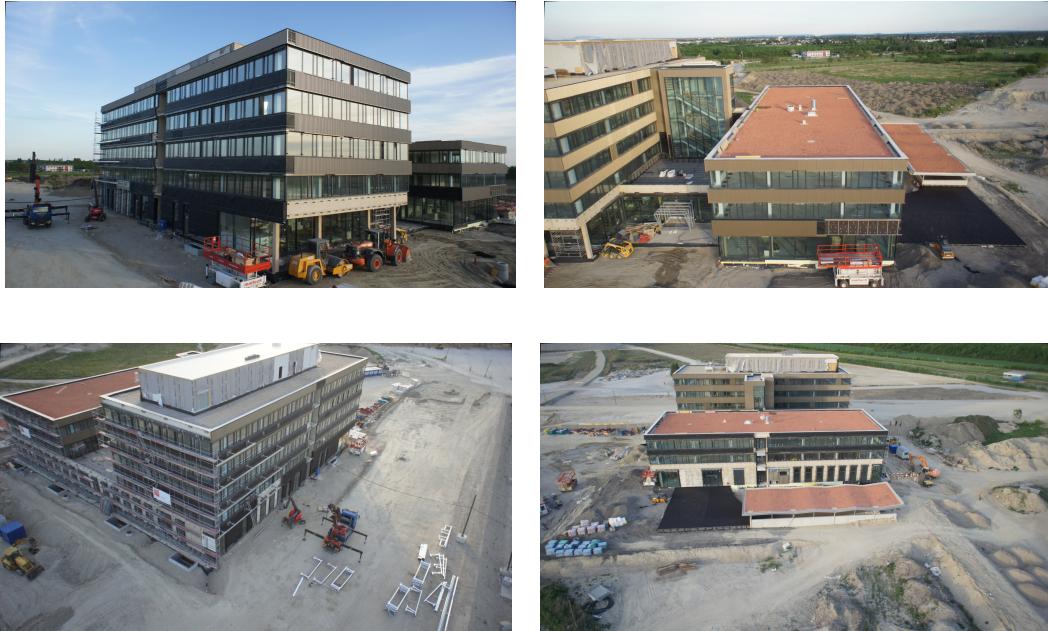
Figure 5.7: Images from Aspern building taken from an UAV. As you can see, it contains many surfaces consisting of glass. Additionally, a part of the roof is completely white, which also leads to clutter in the reconstruction (bottom left image).
