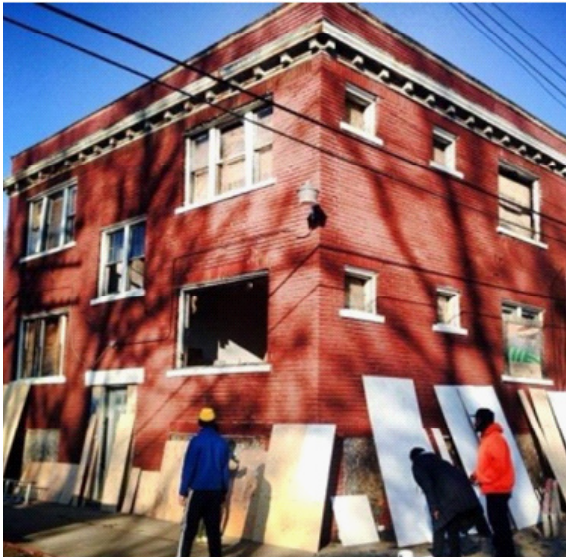
Fig. 97: Community Center - old structure The beginning of the restoration
