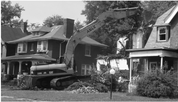
Fig. 68: Demolition of a house in Detroit, North End
