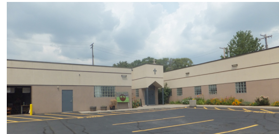
Fig. 76: Earthworks Capuchin Soup Kitchen
