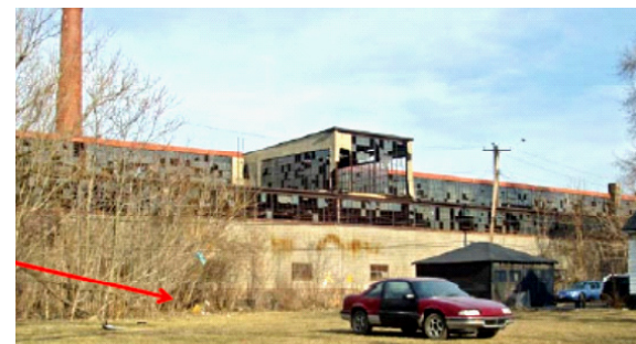
Fig. 65: Illegal parking, unpaved and no parking stripes
