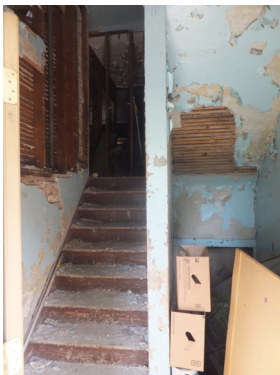
1 Fig. 92: View staircase secondary entrance
