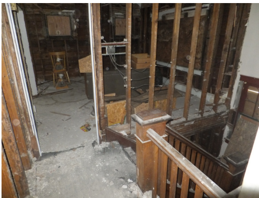
2 Fig. 91: View from staircase main entrance to the room structure
