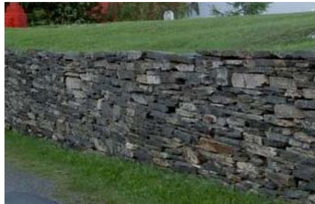
Fig. 2: Rip Rap (Steinwurf) [I] and Dry Stone Wall (Trockensteinmauer) [II]
