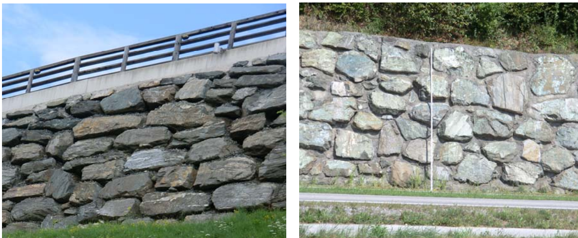
Fig. 20: Stacked and mortared, Natural Rock Wall
