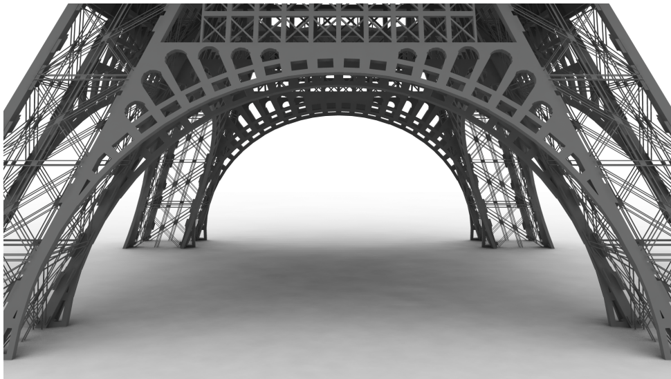
Figure 5.10: One of the decorative arches of the Eiffel Tower, also note the lower platform, and the grid that connects the arches with the lower platform
