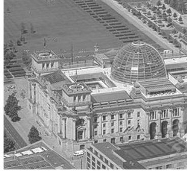
Fig. P. 25 (right): Aerial view of the Reichstag building
