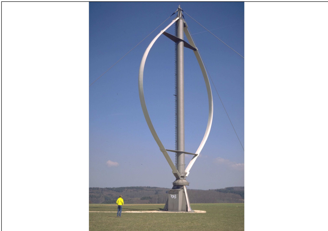
Figure 3.24 : Darrieus Rotor 62
