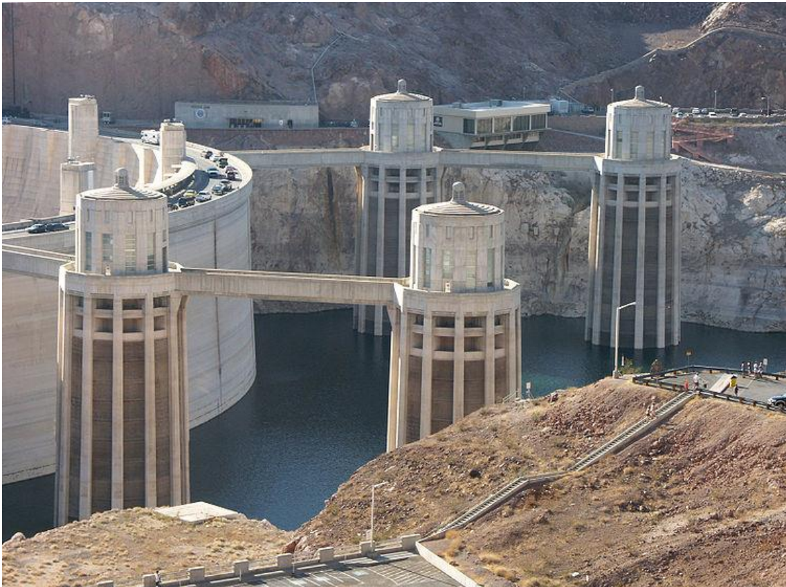
Figure 1: Tower intake at Hoover dam, Colorado River
