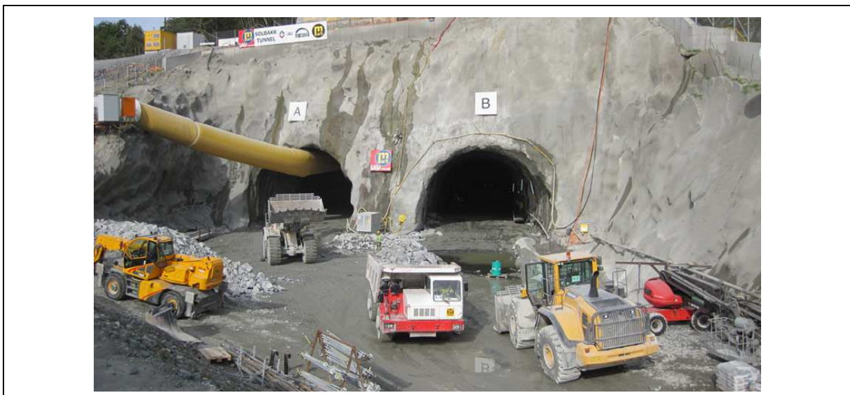
Figure 1: Solbakk tunnel in Tau - Norway
