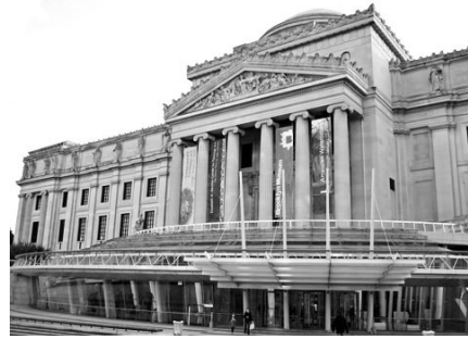
3.109 Brooklyn Museum, Entry Pavilion and Plaza, NY, Ennead Architects, 2004
