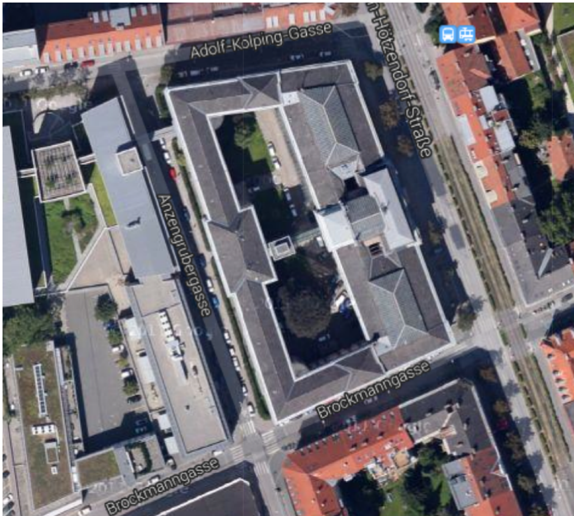
Figure 5.1: Testing area, this is an aerial detailed image of the testing area.
