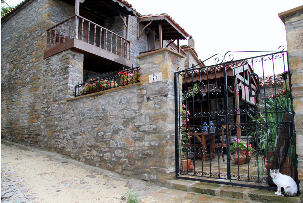
Figure 6: A house in Eski Bademli Village
