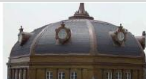
The Roof of one of the Domes (with Japanese Slate)
