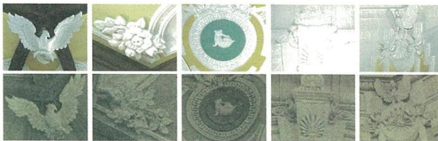
Figure 6.40 Ornamental Details in the Domes – restored (above) and original (underneath). 250
