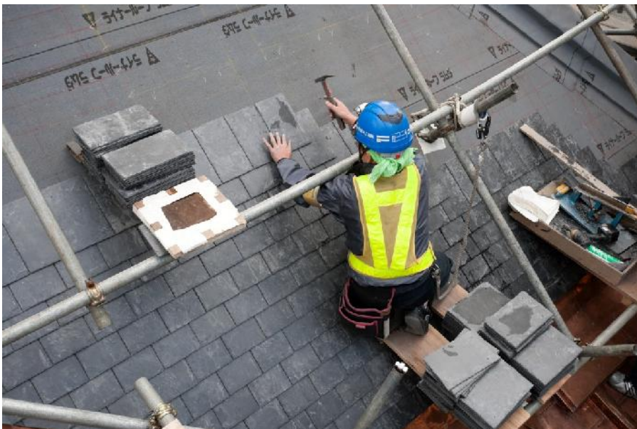
Figure 6.45 Nailing slates. 255
