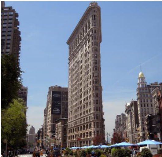
Figure 1.1 The groundbreaking skyscraper “Flat Iron Building”. 4
