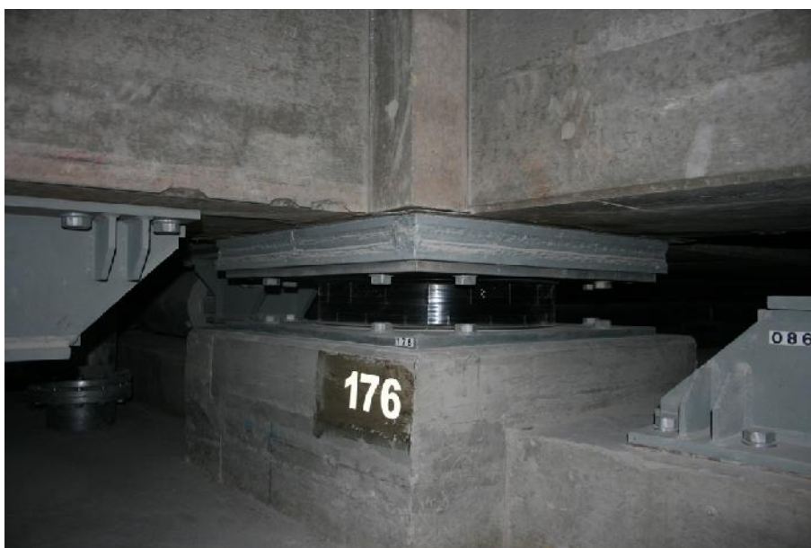
Figure 6.35 Installed Isolating Rubber. 245
