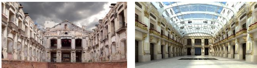
Figure 16 Sofiensaal after the fire 328 and after reconstruction 329
