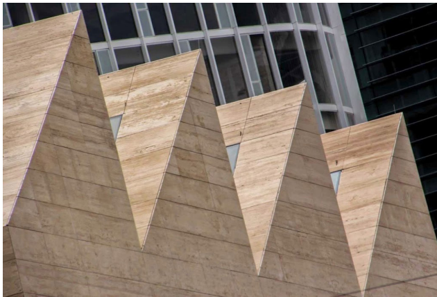
Figure 5-12 - Saw Tooth Roof
