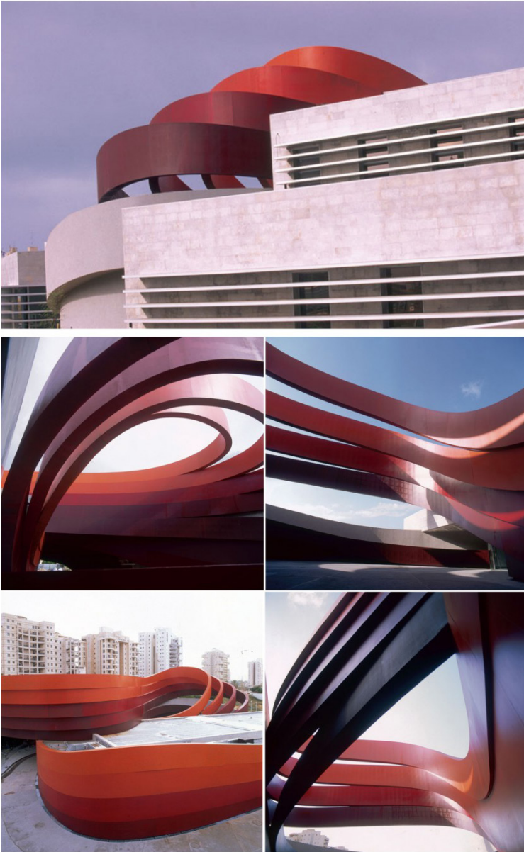
Figure 5-07 - Cor-Ten Steel Bands
