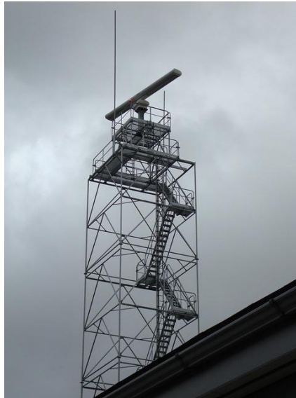
Figure A.1.: A sample SMR installation at Tallinn airport.
