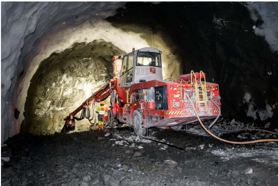
Figure 27: Ongoing drilling process at the face with a Sandvik drilling jumbo
