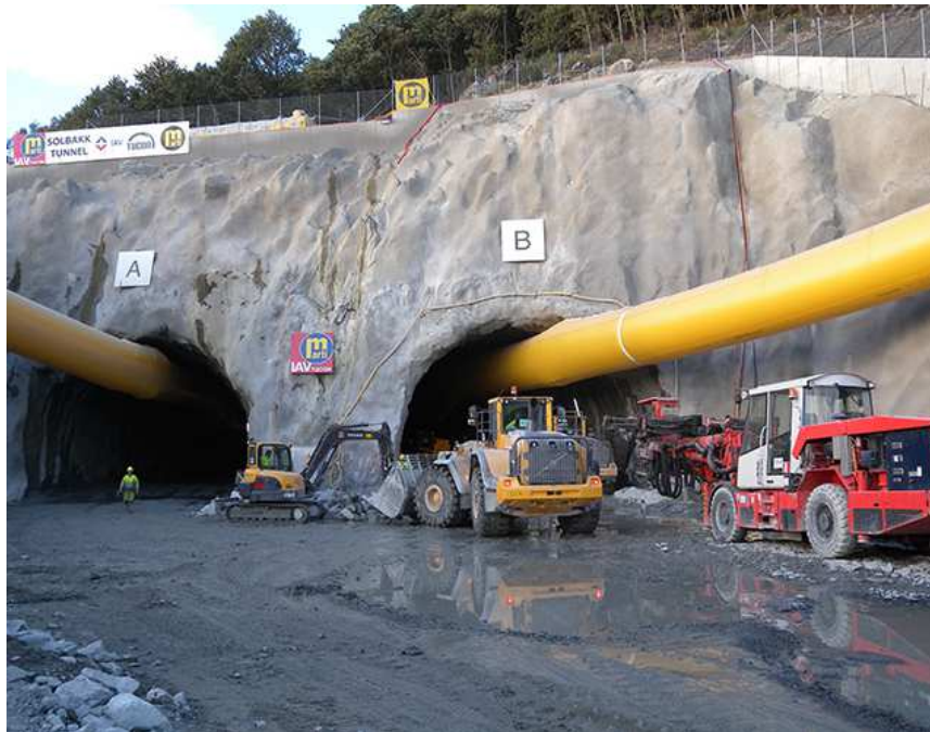
Figure 1: Portal area of the Solbakk tunnel (North side)
