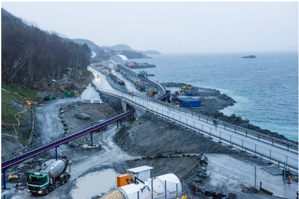
Figure 31: Overview of the construction site Solbakk / Tau
