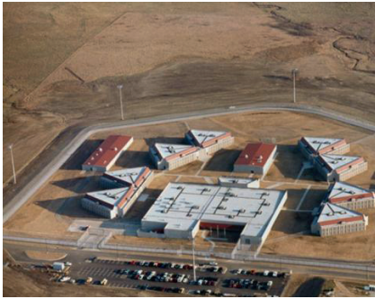
049 davis correctional facility | cca | amerika
