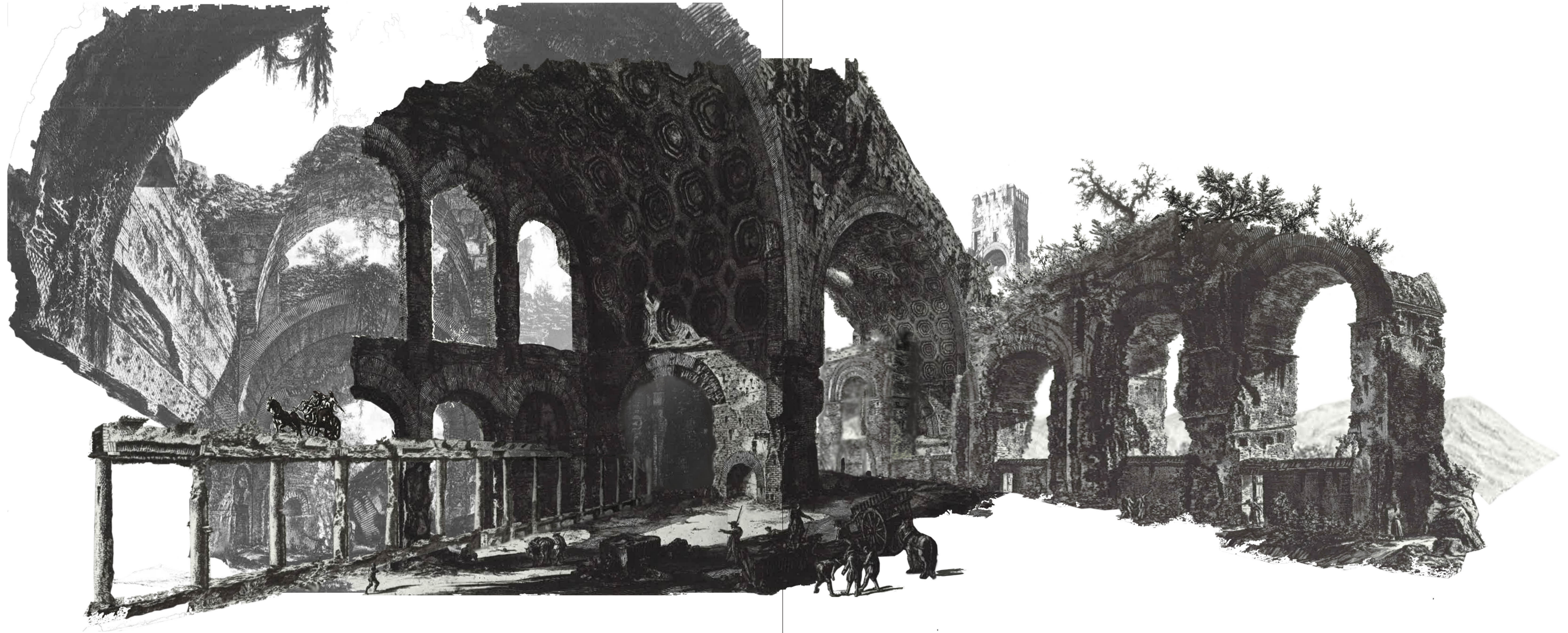
25 this collage represents a mockup of gravures symbolizing some of the ruins of Campo Marzio envisioned by Piranesi, specially selected to suggest the idea of interaction between urban pieces of infrastructures combined with framing
