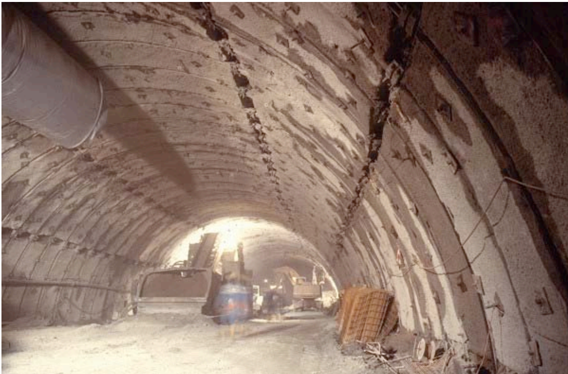
Photograph 1.: Inntal tunnel_Excavation in heavily squeezing rock 1
