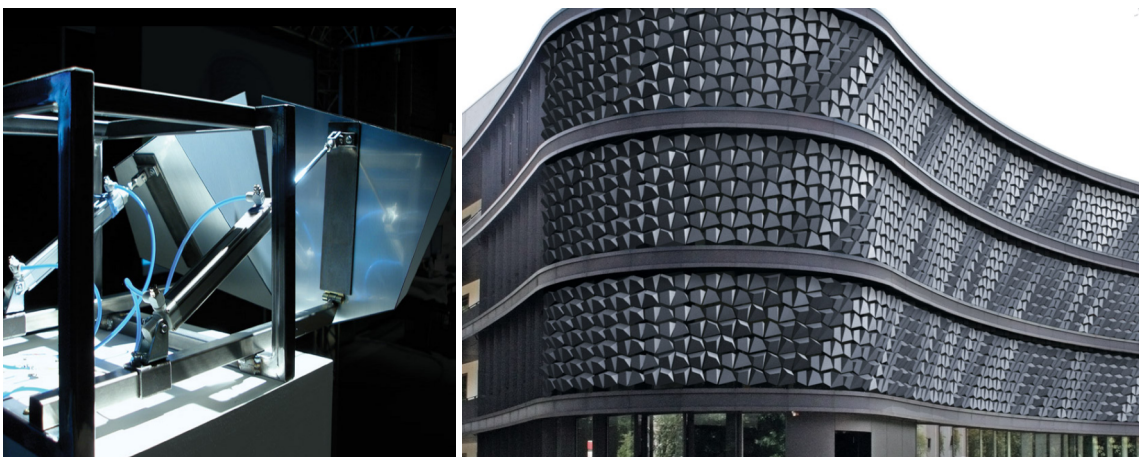
Figure 2.5: The flare display from behind with pneumatic actuators and mounted on the façade (from www.flare-facade.com/ ).
