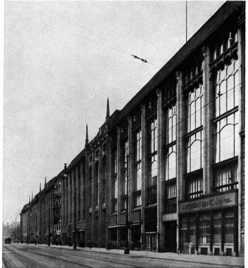
394 / BERLIN Warenhaus Wertheim Department Store Anbau in den Formen Messels
