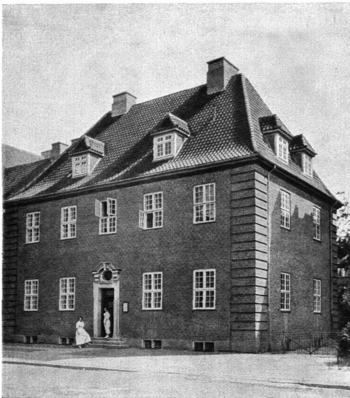
238 / COPENHAGEN Sjoellandsgade. Badeanstalt Municipal Baths Designed by the City-Architect
