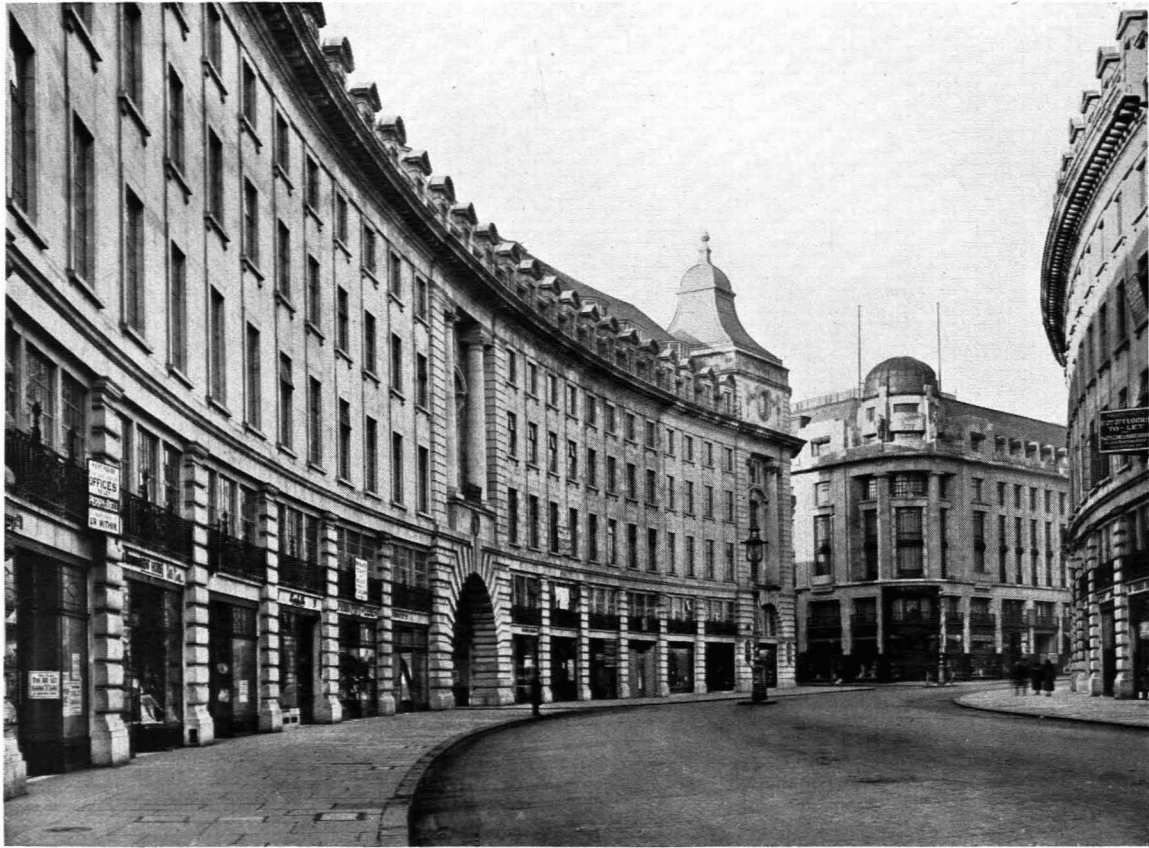
141 / LONDON Regent Street. The Quadrant. 1926. Arch.: Reginald Blomfield, Aston Webb, Ernest Newton
