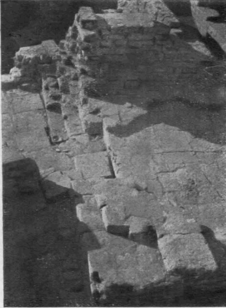
Abb. 22: Genutete Dilatationsfuge am Ishtar-Tor.
