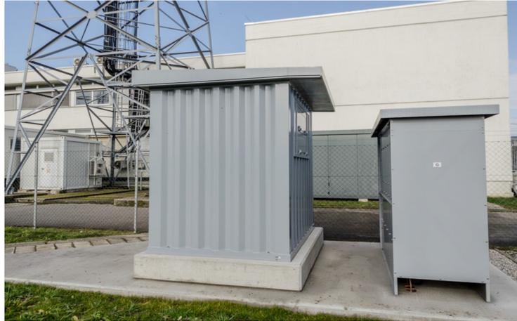
Figure 24: HPE resistor (right hand side) and switching logic (on the left) as published in [37]
