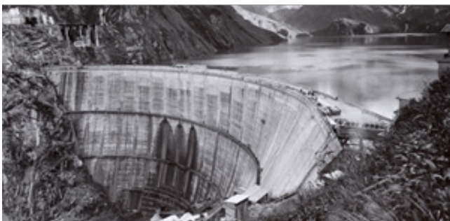
Construction phases of the Limberg dam [ 5 ]
