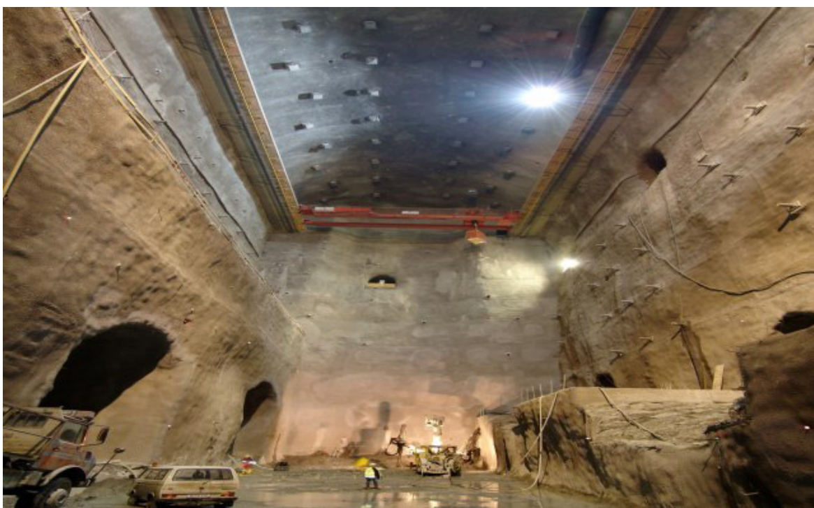
Construction site of Kopswerk II cavern [ 2 ]
