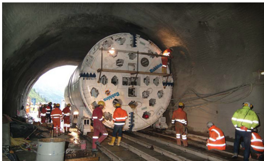
Construction site of the headrace tunnel Kopswerk II [ 5 ]
