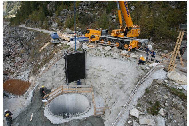
Construction site at the reservoir Wurten in 2007 [ 1 ]
