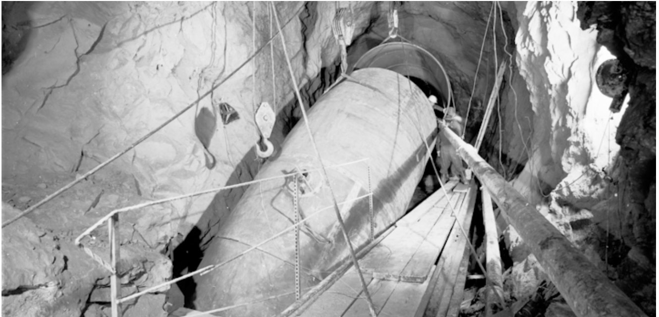
Headrace tunnel Roßhag under construction [ 3 ]
