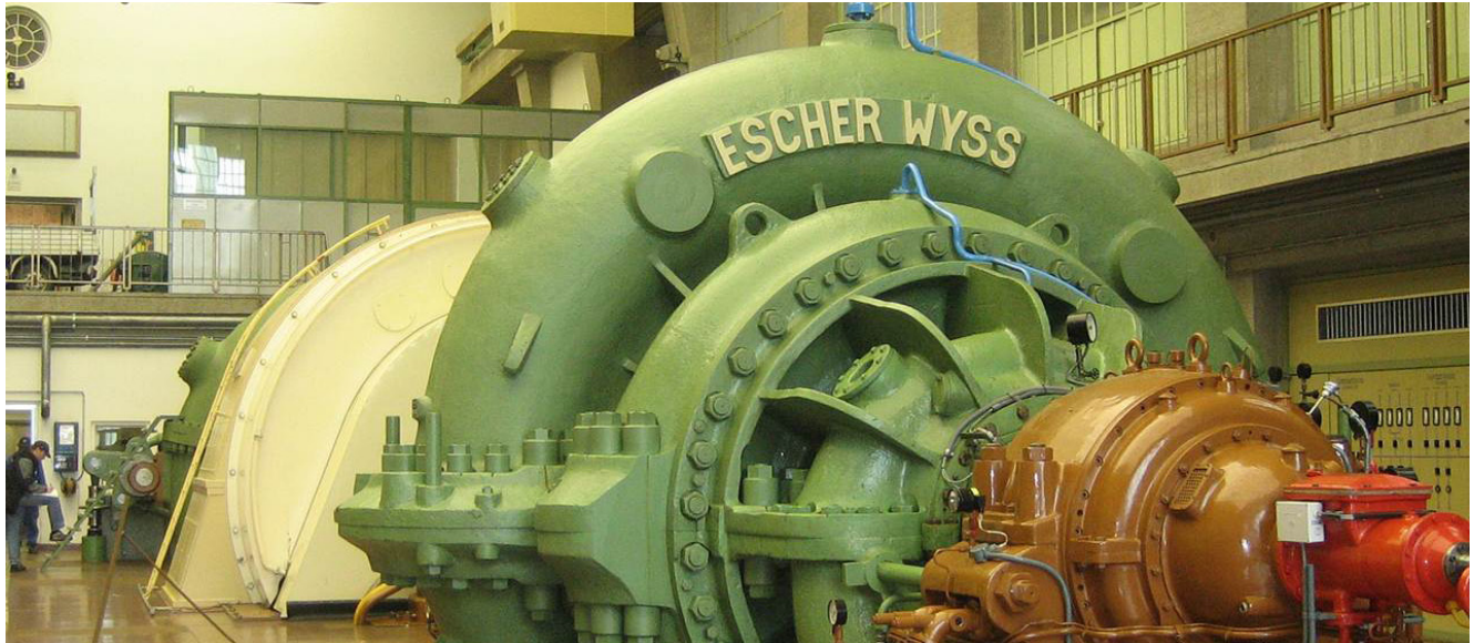
Ternary machine unit of Limberg I [ 5 ]
