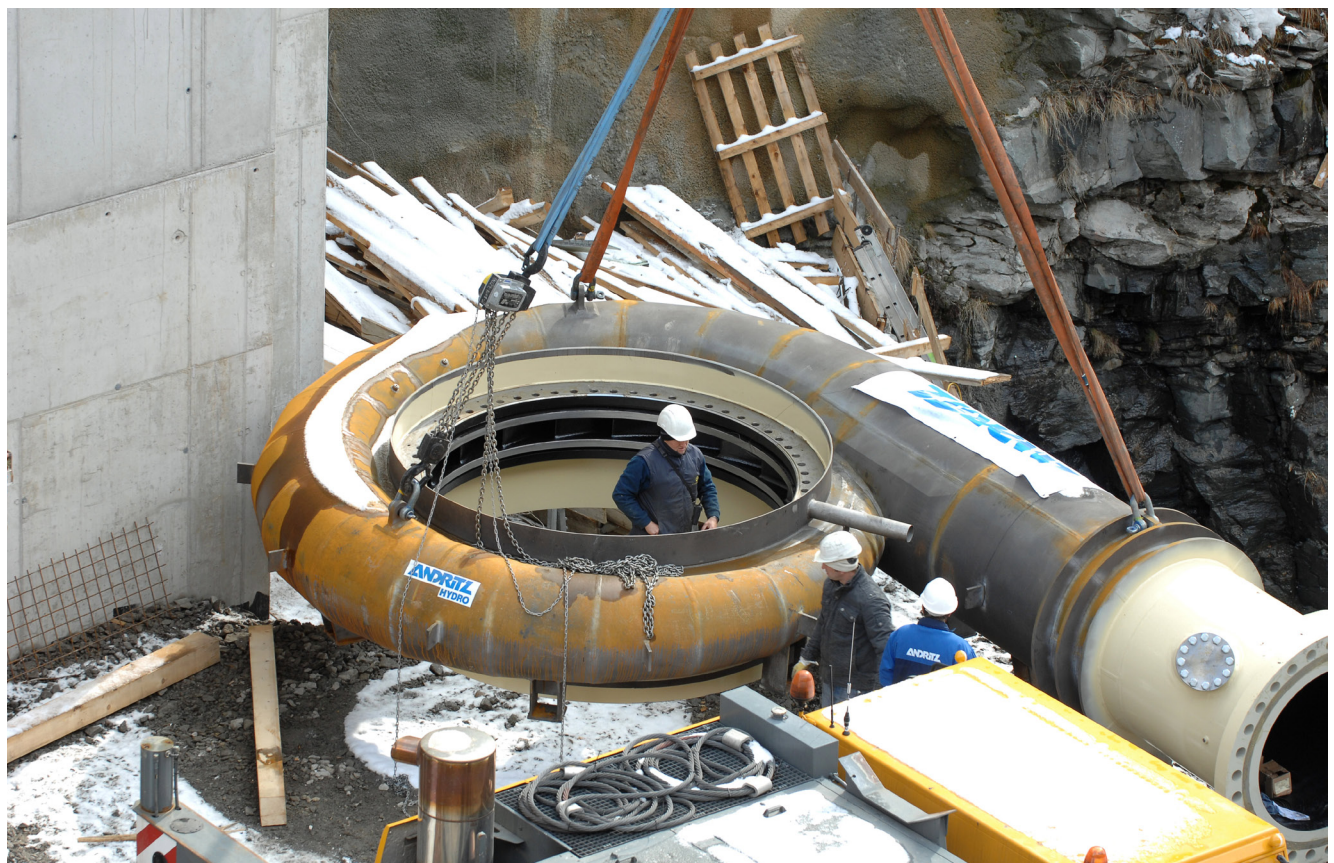
Positioning of the spiral in 2010 [ 1 ]
