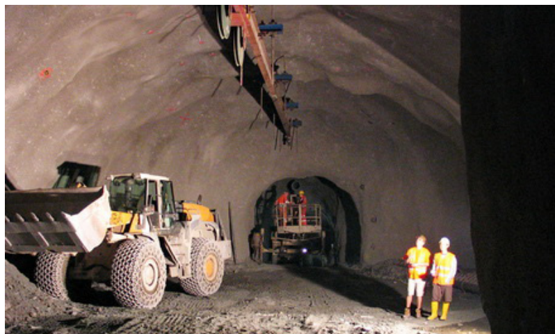
Construction site at the headrace tunnel [ 12 ]
