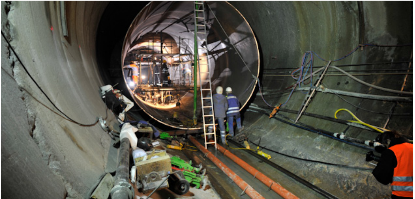
Construction of the headrace tunnel of Limberg II [ 3 ]
