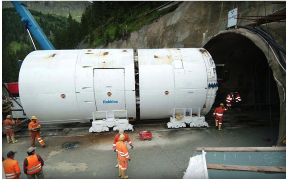
The Robbins TBM at Kopswerk II [ 5 ]
