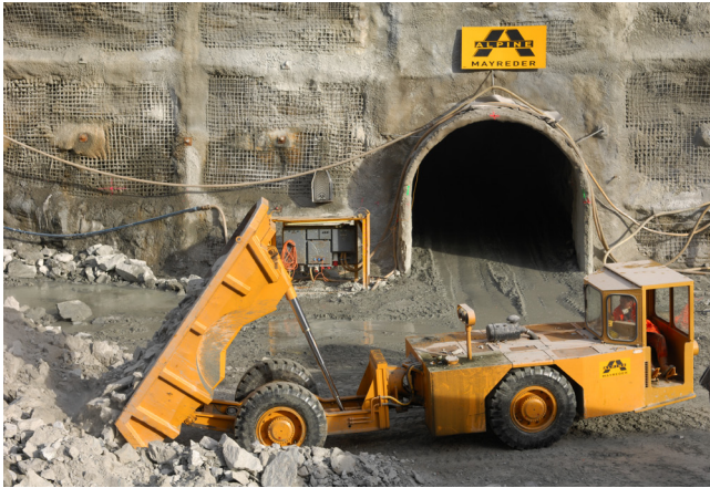
Adit portal in 2007 [ 1 ]
