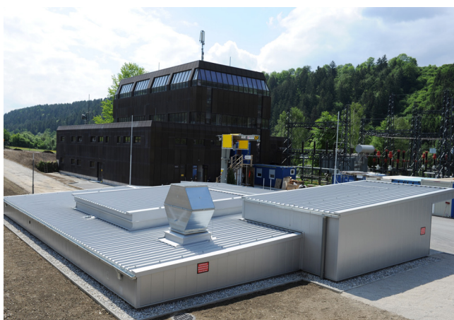
Pump shaft Koralpe [ 4 ]
