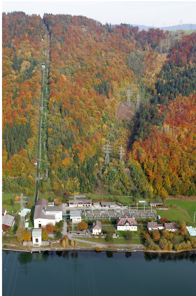
Aerial view of the power station Ranna and the pressure shafts [ 1 ]
