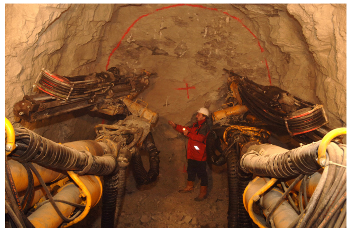
Monitoring in the tunnel in 2006 [ 1 ]
