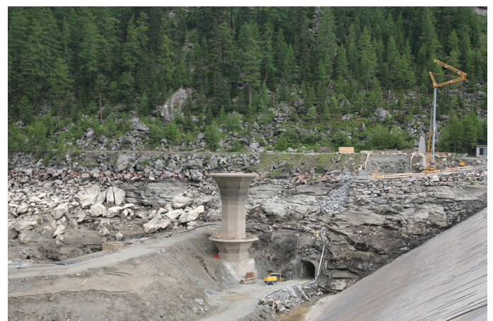
Reservoir Wurten during construction in 2007 [ 1 ]
