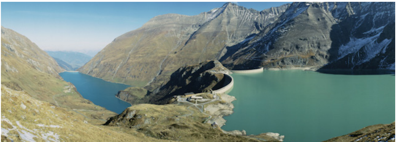
Kaprun Upper Stage - Mooserboden and Wasserfallboden reservoir [ 5 ]
