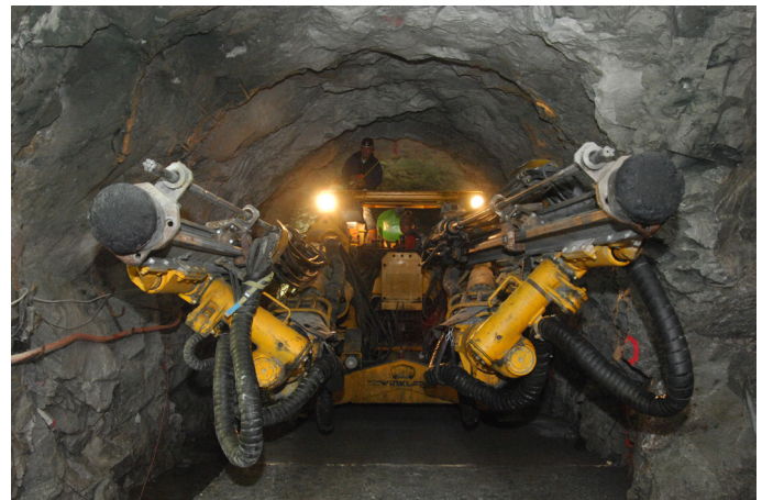
Drilling jumbo at the tunnel in 2006 [ 1 ]
