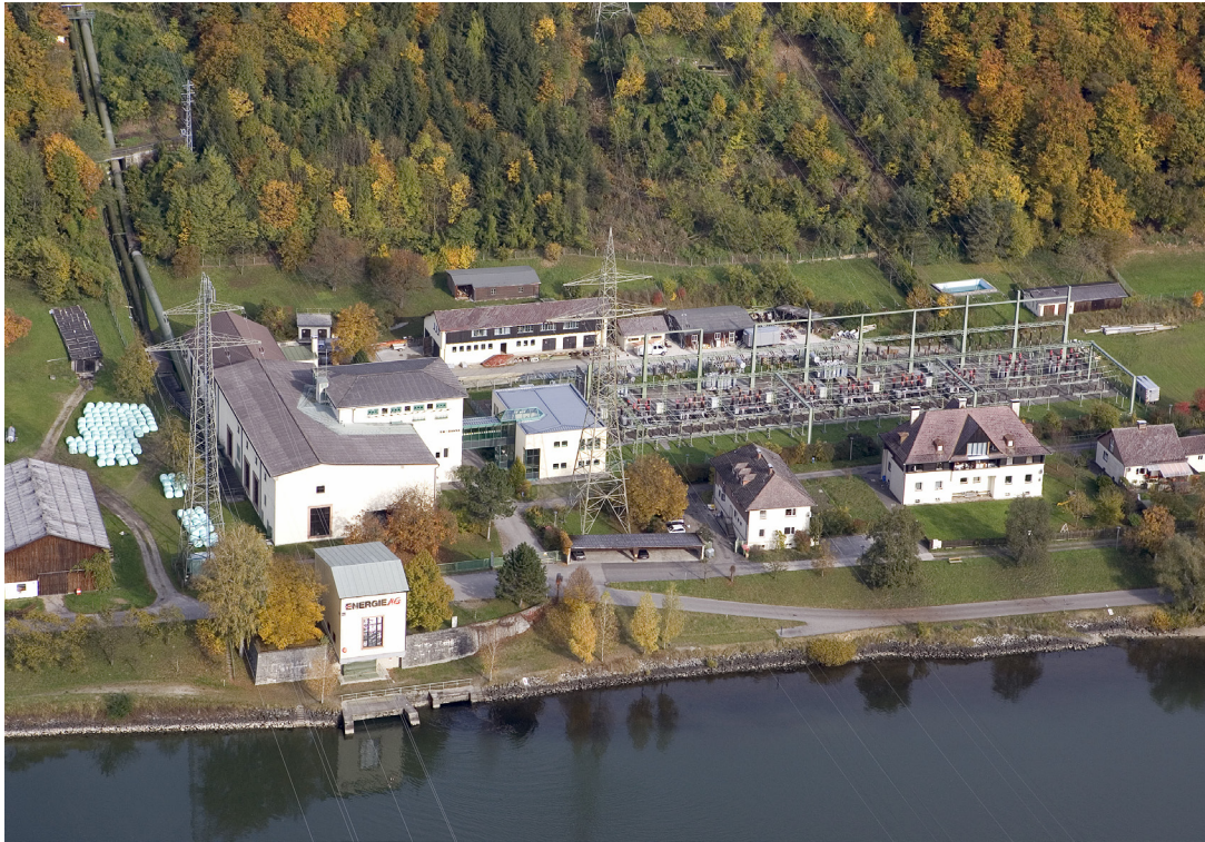
Aerial view of the power house Ranna and the switchyard [ 1 ]
