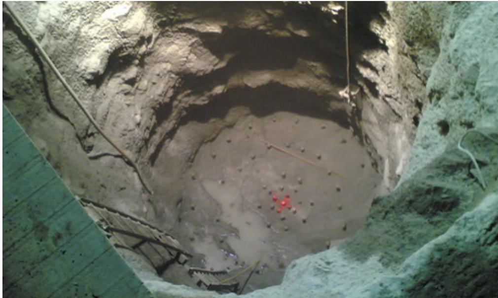
Bottom of the rising shaft [ 8 ]
