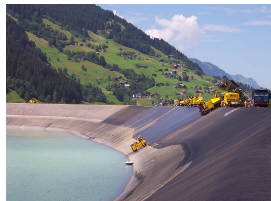
Extension works at the Rifa reservoir [ 3 ]
