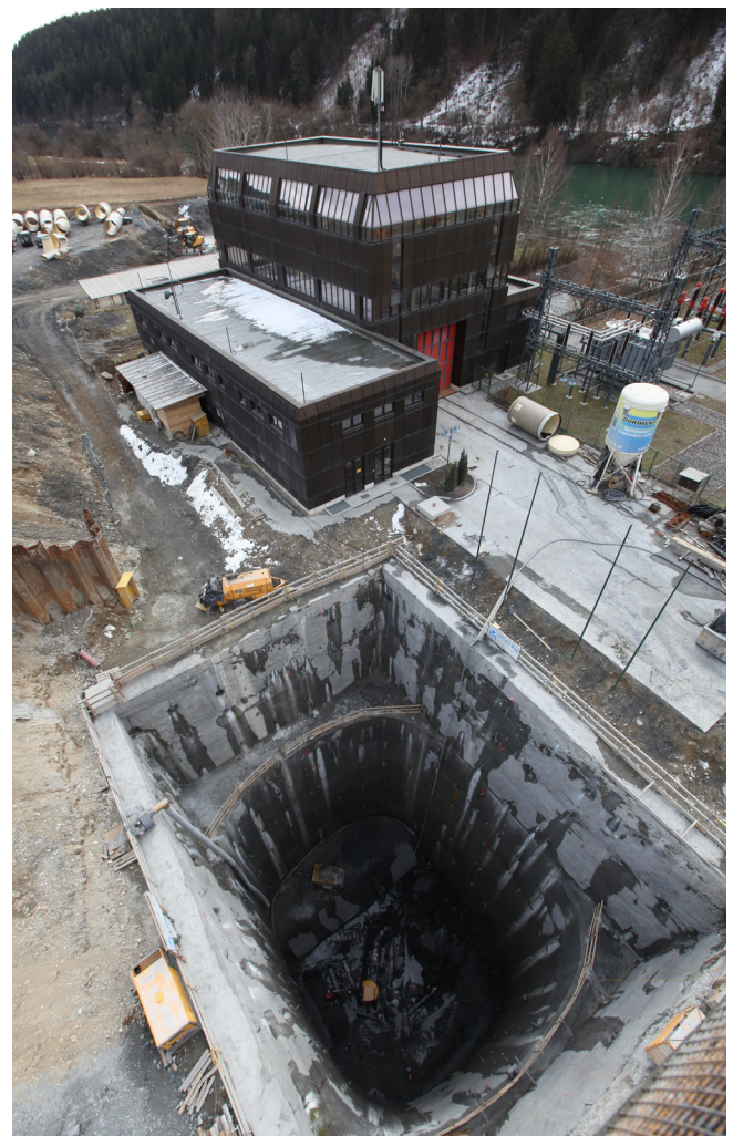
Pump shaft Koralpe under construction [ 4 ]
