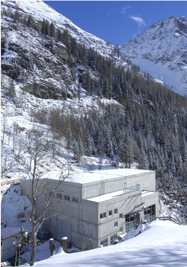
Power house Feldsee in 2011 [ 1 ]
