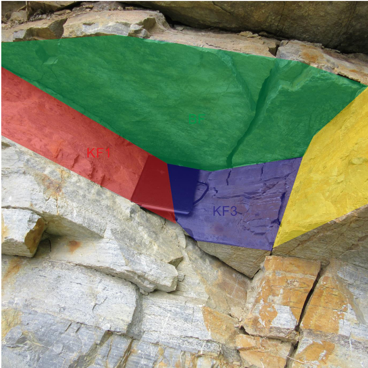
Figure 44: Mould 2 (Oberwölz), showing all joints and free planes.
