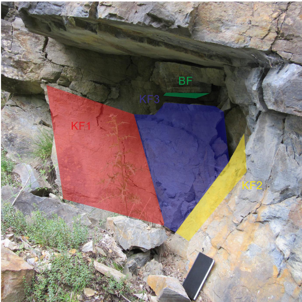
Figure 40: Mould 1 (Oberwölz), showing all joints and free planes.
