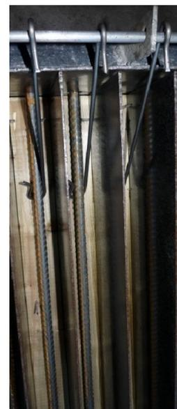
Abb.6 Shear - Connector
