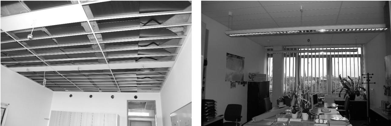
Figure 1: Installation of the PCM-boards in the ventilated cooling ceiling (left) and built-in sun protection system with PCM (right).
